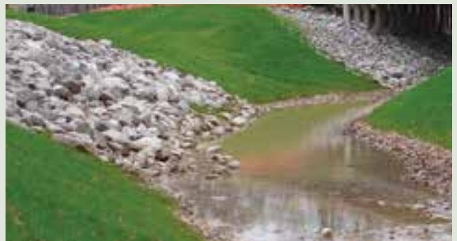
WATERWAYS: The ideal solution to stabilize banks where heavy rain is expected, and resolve other environmentally sensitive challenges.
