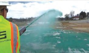
FINN invented the HydroSeeder® in 1953 creating a new industry of turf and erosion control contractors. Hydroseeding is far more efficient than broadcast seeding or installing sod. It speeds the seeding process, saving time, labor hours and money. And the results are lush, thick grass beds that establish quickly.
