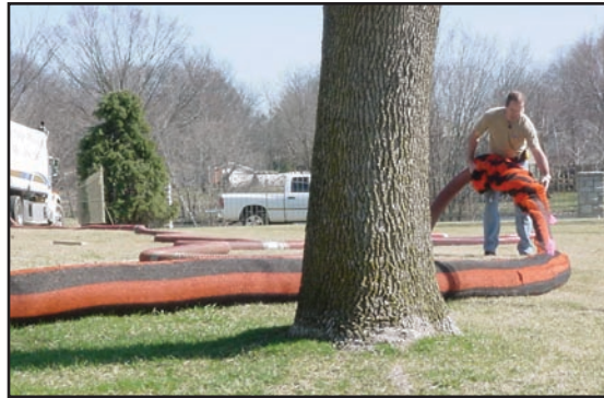
Installation Method – Perimeter Control
