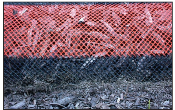
Close Up of Sediment Control
