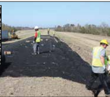
US Army Corps of Engineers Levee Construction
