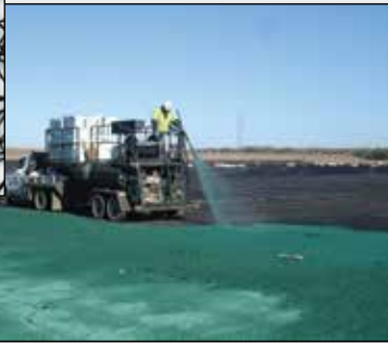
Flexterra® HP-FGM™ applied into TRM 7003
