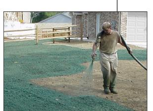
In many segments of our industry, the demand for applications that require the pumping of heavy, dense slurry materials has driven the developments of various pump alternatives. Projects that are requiring these intense applications are golf course turf establishment, spray-on erosion control, landfill covering and sod field establishment. The materials that are used on these jobsites can be as unique and variable as the applications themselves.
