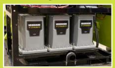
Powered by 3 Vanguard 5kwh, 48 VDC, Lithium-Ion Batteries in parallel.
